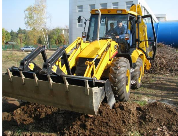
Buldoexcavator JCB 3CX – lucrări practice
