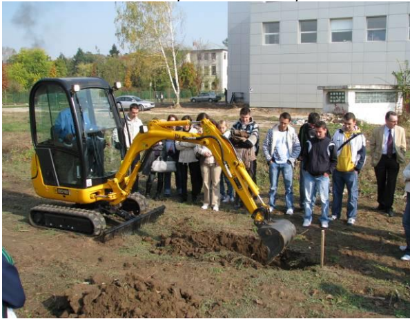
Miniexcavator – lucrări practice
