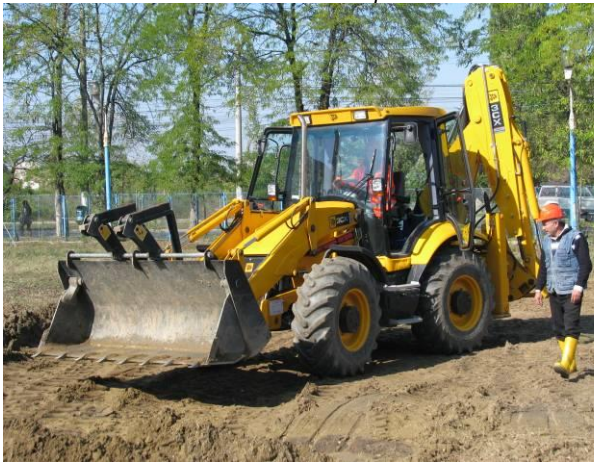
Buldoexcavator JCB 3CX – lucrări practice
